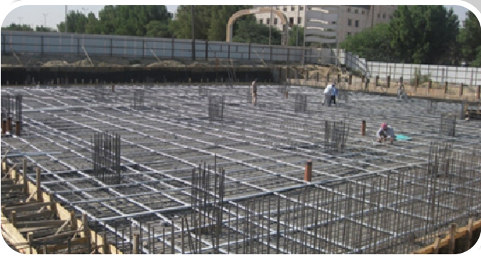
Bonded PT Slab
